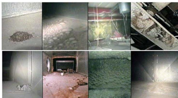
Fig. 2. Contamination in supply and return ductworks.
